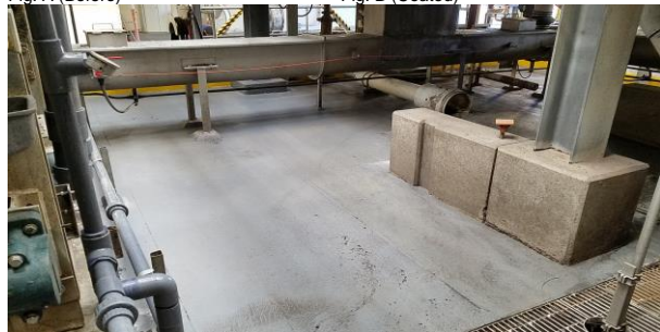
Fig. C (2-Years later) No blistering or delamination on impact zones
